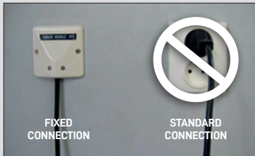
FIXED CONNECTION (HUBER 360® EVOLUTION) AND STANDARD CONNECTION (PROHIBITED)
